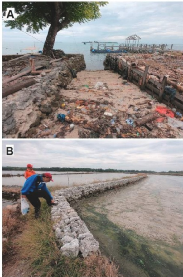
Fig. 2. A. Coral rubble employed to reinforce coastal walls, and B. Dead corals employed to build walls of aquaculture ponds. Both photographs taken by Sarah Hamylton at Sabangko Island, July 2019.
